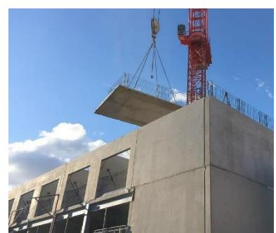
high-quality finish of pre-cast components can be combined with the economy and flexibility of cast in-situ concrete.”
