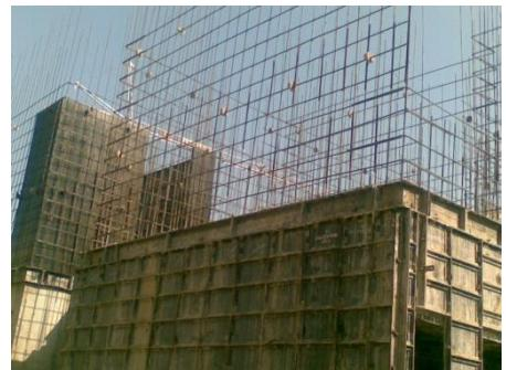
100 mm thick RCC walls and slab have thermal transmittance (U) value of about 3.6 W/m<sup>2</sup>K). As, it is more than the normal plastered brick masonry walls (U= 2.13 W/m<sup>2</sup>K), it is advisable to ensure proper planning for heat insulation and air ventilation in the housing units.
